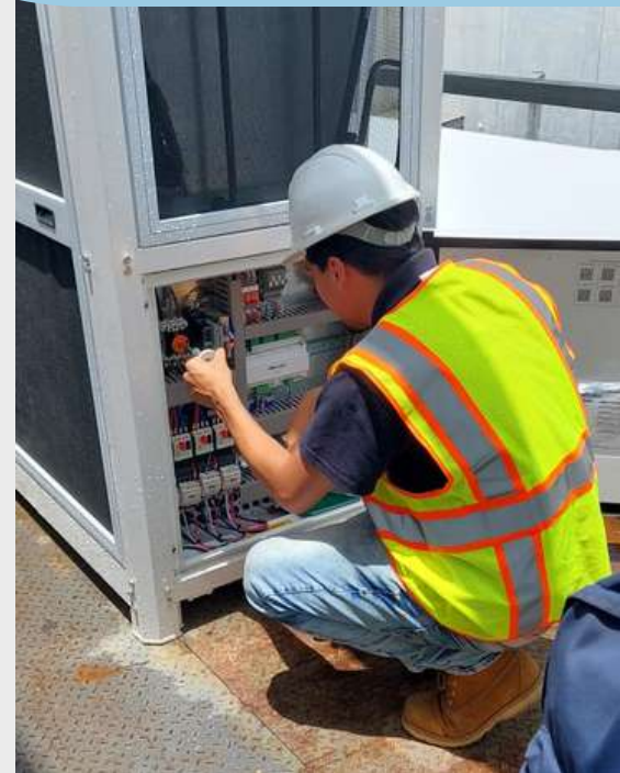
Service on a Mecalor chiller
